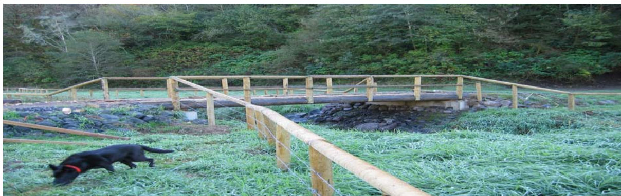
Upper Johnson Fence and Johnson Bridge #1
